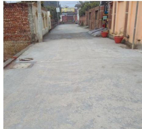
Work done in Ganpati Enclave
